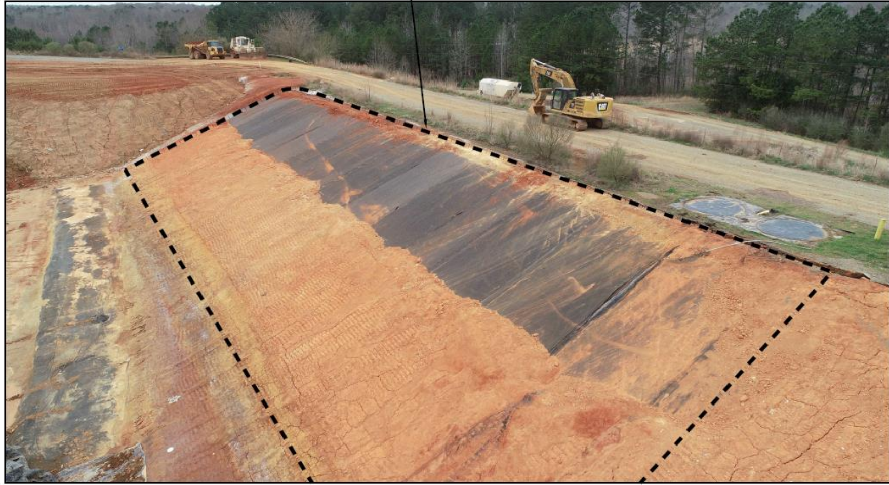
WEST OF PUMP RISER SHORTLY AFTER RAIN COVER REMOVAL
