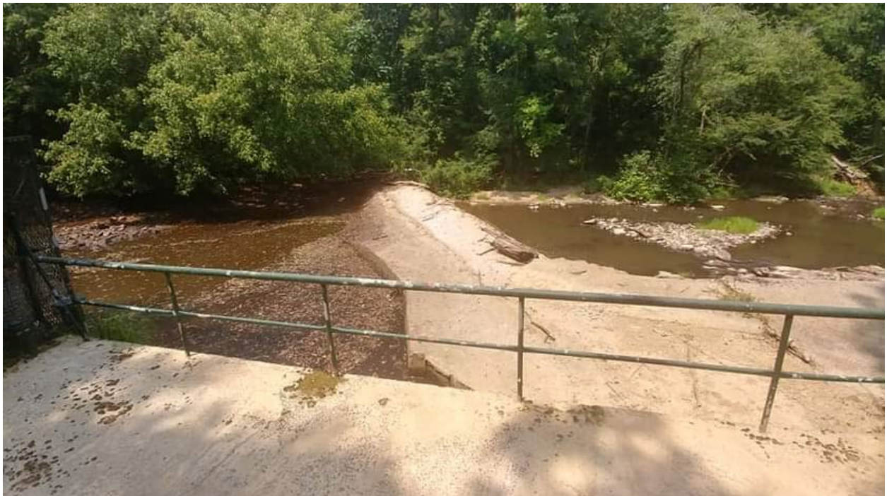
Dam at the Mill Pond, Behind Guthrie Mill
